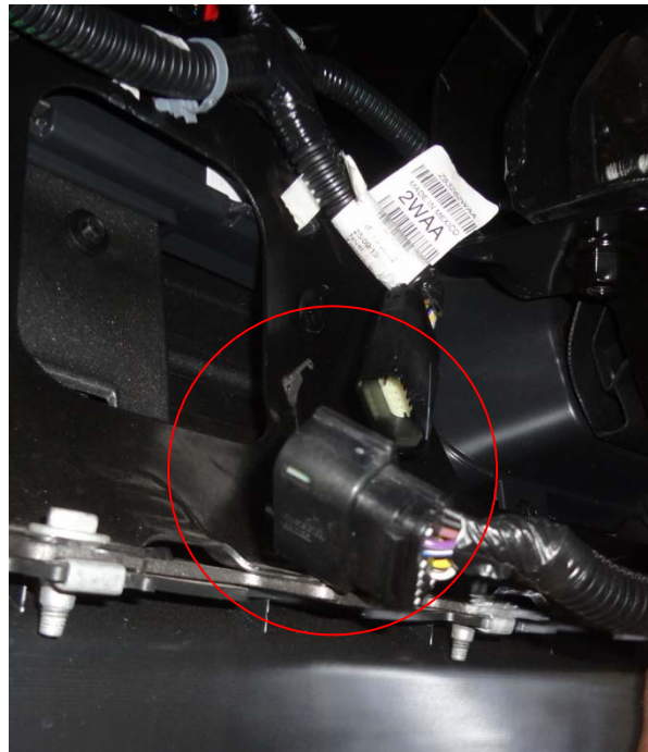
Figure 3(electrical harness disconnected)
